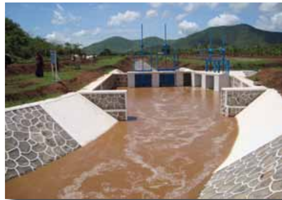
Figure 7: Bifurcation structure of pump canal and weir right main canal
