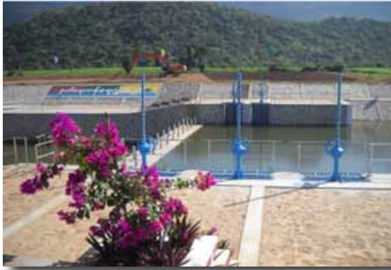
Figure 5: Weir structure, head regulator and silt excluders of Shwe Hlan Bo Region Greening Project
