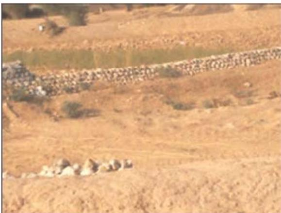
Figure 5. Tihama, Yemen: stone-pitch overflow control structure
