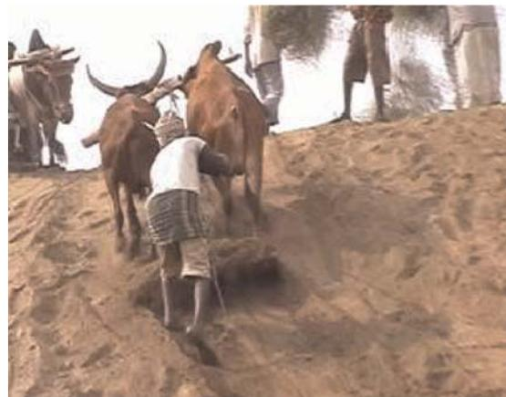
Figure 4. Wadi Laba, Eritrea: field bund maintenance with oxen-driven *mejhaf*
