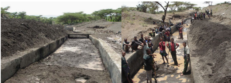
Fig. 5 Sedimentation problem in Fokisa, Tigray, Ethiopia (Gebreegziabher Embaye et al. 2008)
