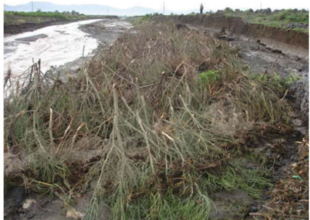
Fig. 3 Traditional diversion structures in Hara, Tigray, Ethiopia (Haile 2009)
