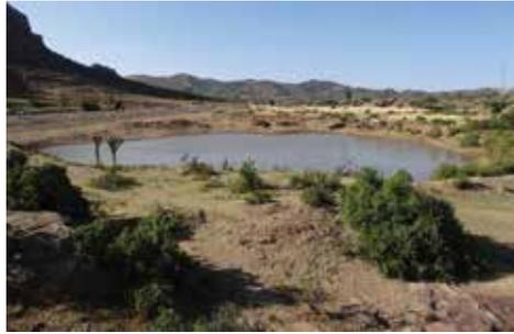
**Figure 2** Pond used to harvest runoff from culverts for livestock and groundwater recharge in Wukro area, Tigray, northern Ethiopia
