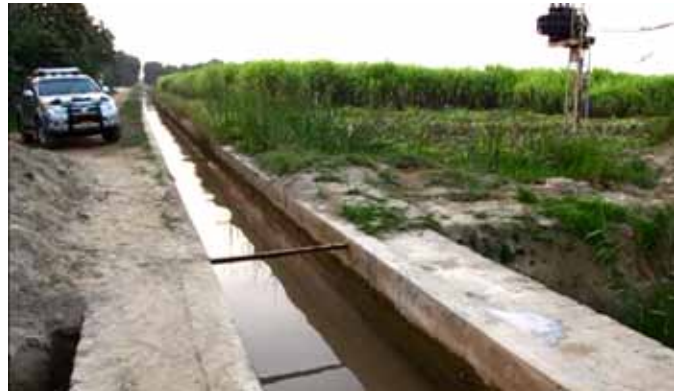
Figure 9: In Tandoallahyar, farmers decided to line their watercourse to prevent seepage and waterlogging.
