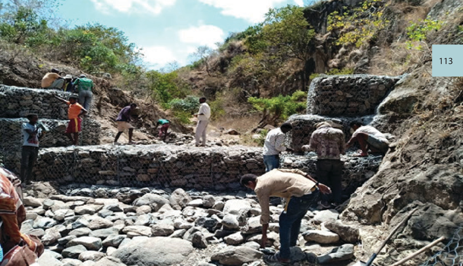
Gabion check dam constructed in Biskelo river, Soke Bokicha
